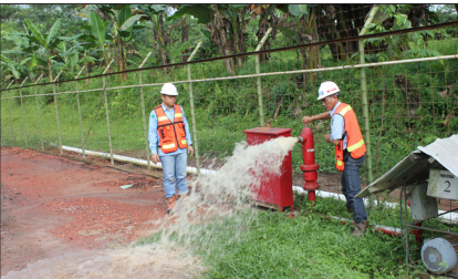
Fire fight safety and management
